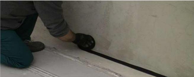
**2** Lay points of a gypsum-based glue on the ground panel or use a low-expansion polyurethane glue
