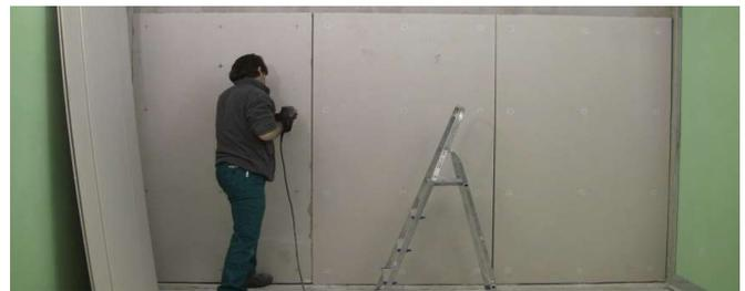
**5** Fix the second gypsum board with the glue and/or appropriate screws
